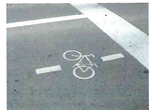
These markings indicate the presence of in-pavement loop detectors that trigger a green light when a bicyclist places their bicycle nearby.
