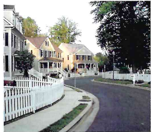
On this residential street, traffic volume is low and cars travel at a slow speed. Bikes and cars can share the travel lane, and there is a sidewalk for pedestrians on one side of the street. (Photo credit: Flickr, Complete Streets Coalition)
